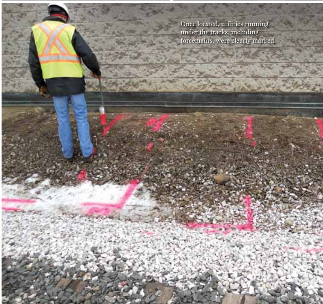
During the GO Transit expansion, the SUE process was implemented to get an accurate depiction of all existing public and privately owned utility services including gas, hydro, water, fibre optics, telecommunications, and signal cabling.
