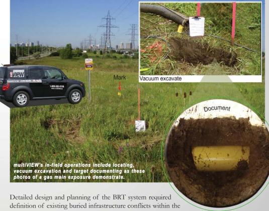
definition of existing buried infrastructure conflicts within the proposed right of way; a major challenge for a project this size. multiVIEW was retained to complete a subsurface utility mapping study following the ASCE 38-02 process which is currently the industry standard (see sidebar on CSA S-250).
